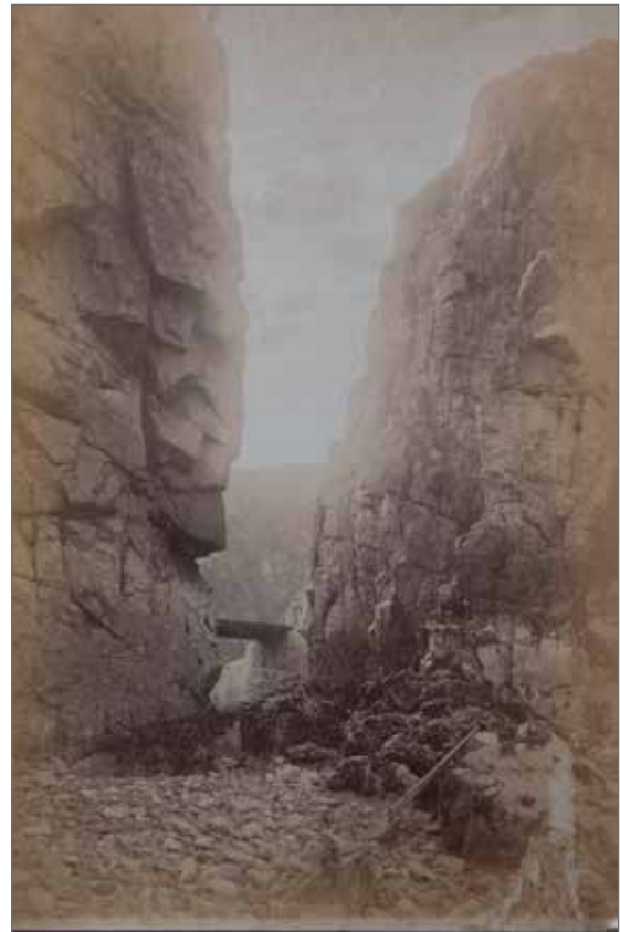
228 Bridge and Rocks, Creux Harbour, Sark 856A1171.jpg T. Singleton Donated by Mrs V Tonks, 1978
