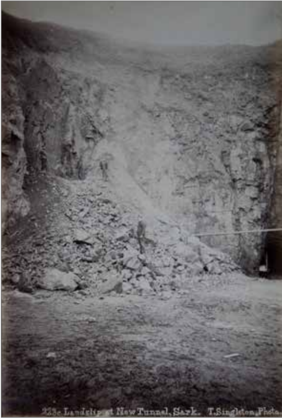
223c Landslip at the New Tunnel, Sark 856A1125.jpg T. Singleton Donated by Deryck Hamon, 2025
